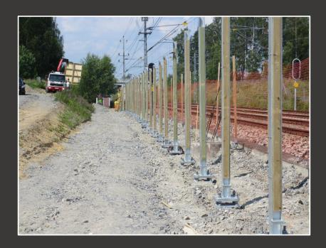
For heavier foundations, the pike is secured in the foundation when the foundation is lying on the ground. The plate lock is then secured in a wing and the foundation is lifted into place.
